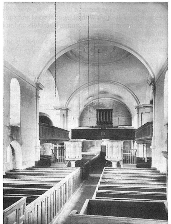
Fig. 4. Dorset, Portland, St. Georges Church, Interior looking west.
