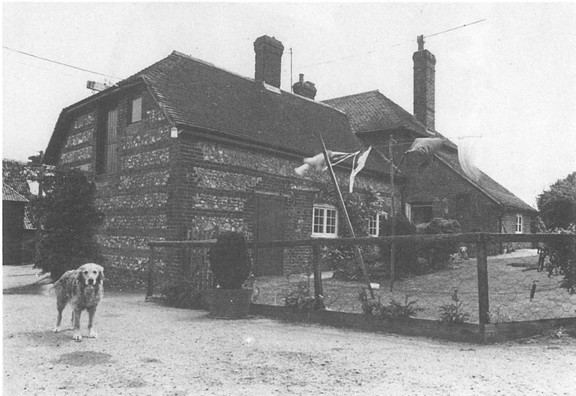
Fig. 3. The banded brick and flint farmhouse at Sutton Hill Farm, now farmed by Mr. Richard Woodhouse, Huxtable's Hill Farm. Copyright Colin Graham, Dorset Magazine.
