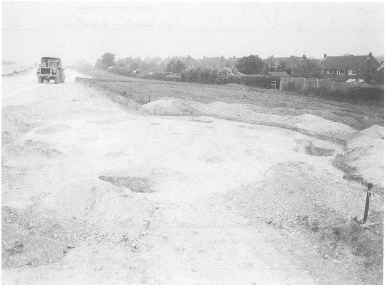
Plate 5. East 'pit ring' fully excavated during by-pass construction.
