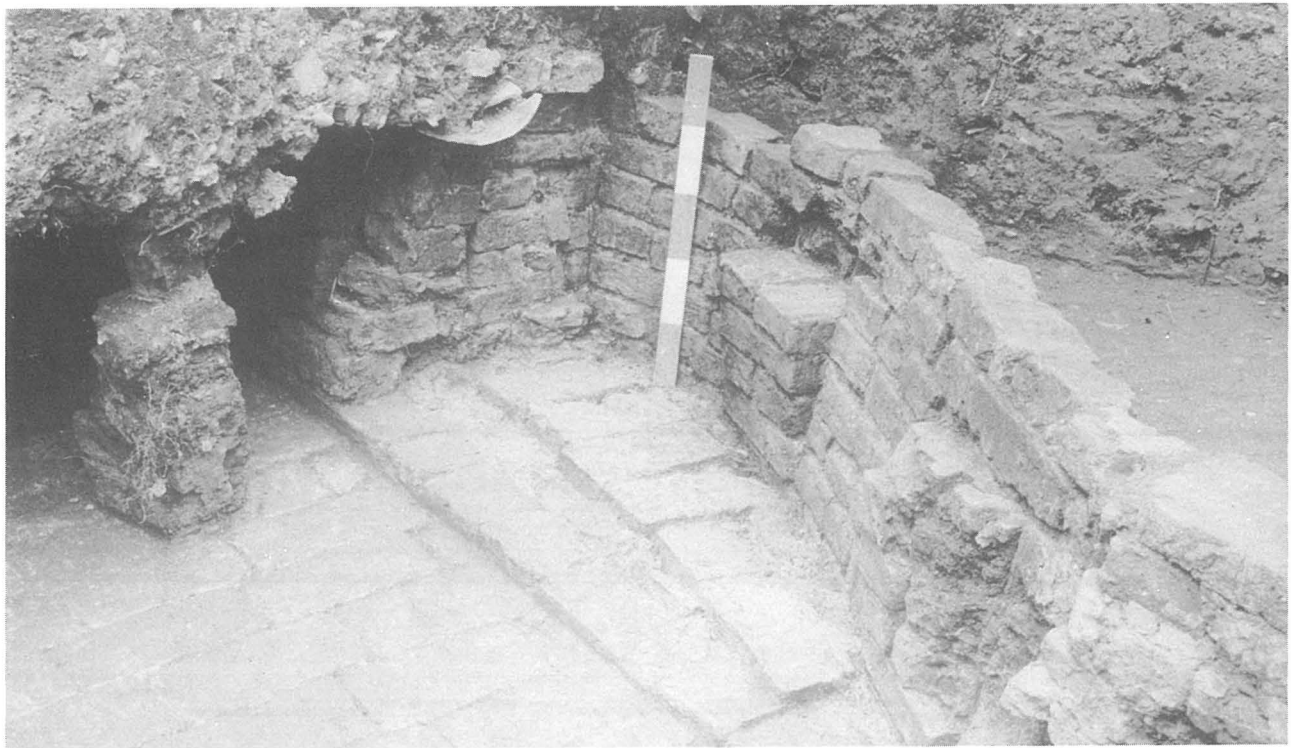
Plate 5. View of chamber from south east with inner skins removed.
