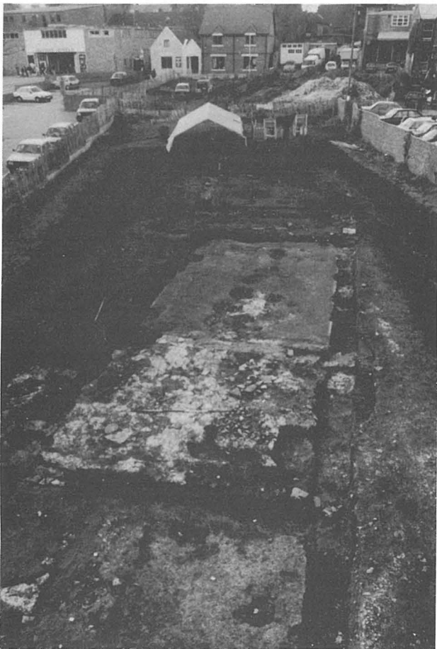
Plate 1. The Charles Street, Dorchester, excavations looking west from Acland Road.
