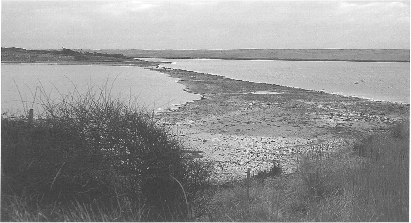
Figure 2: The remains of the Herbury wall
