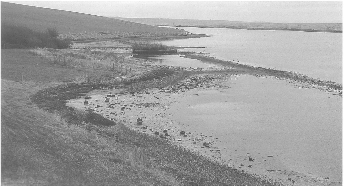
Figure 4: The earthworks in the Fleet below Fleet Manor
