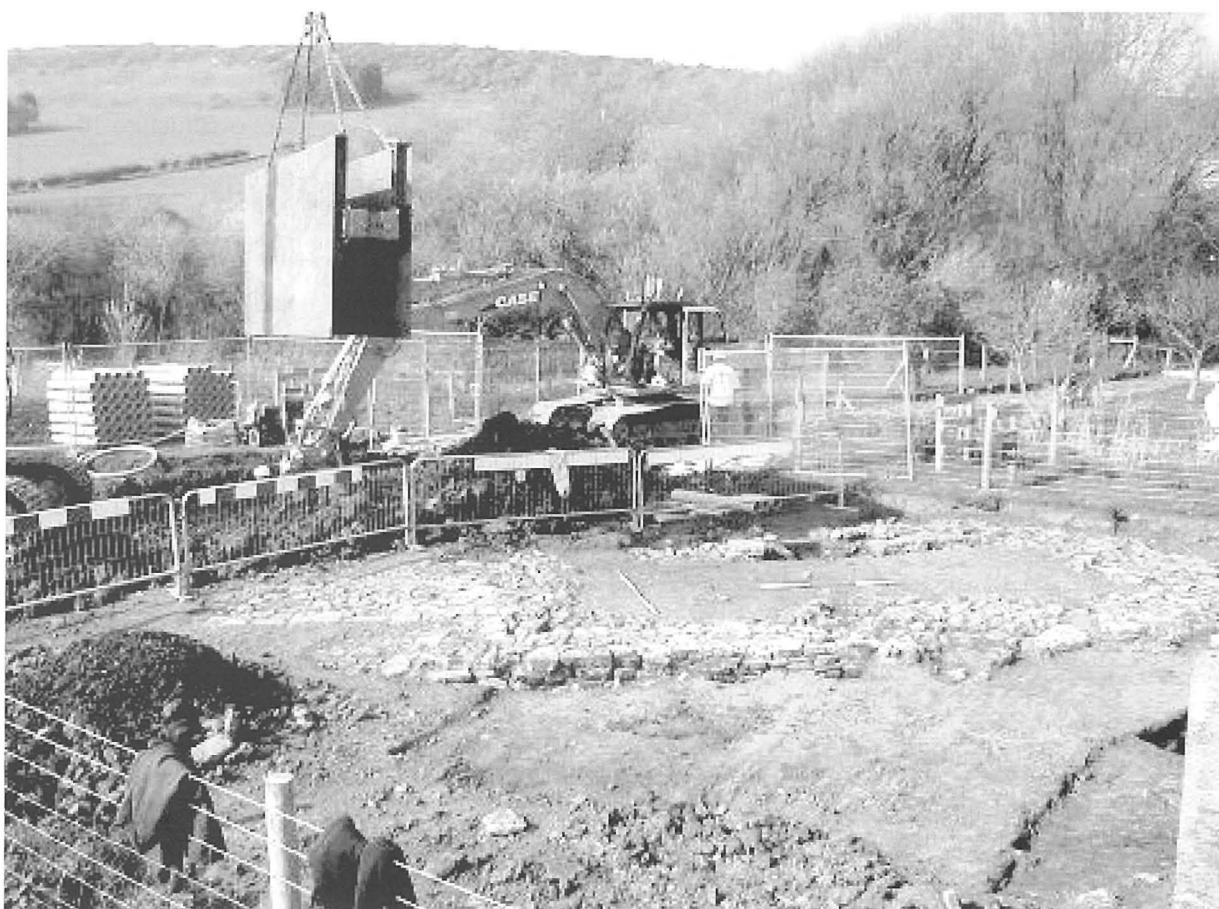
Plate 1. Structure 16, view from south (scales are 2m)
