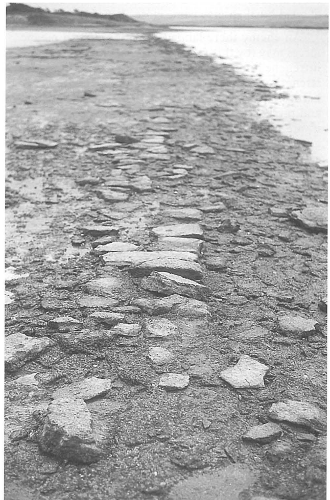
Figure 3: Detail of the Herbury wall
