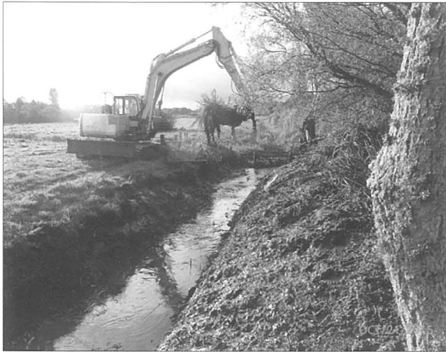
Figure 2: Dredging just upstream of Site 5
