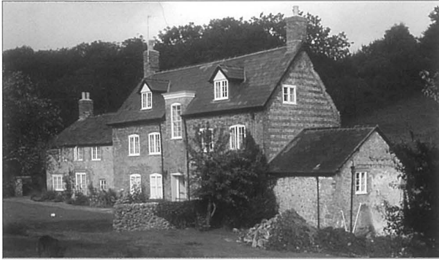
Figure 1: Woolcombe farmhouse south elevation, 1997, showing (to the right) the single storey byre with white painted wall-scar that denotes the area that was shared with the demolished bottling plant (Bournemouth University)
