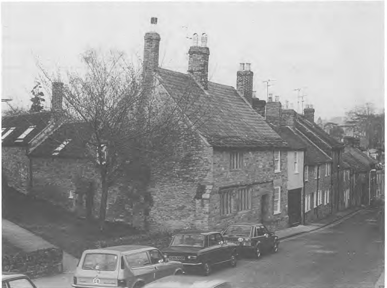
Figure 1. Hall House, Newland, from the south-west after its renovation. Note north-west wing and double doors of passage with loft over.
