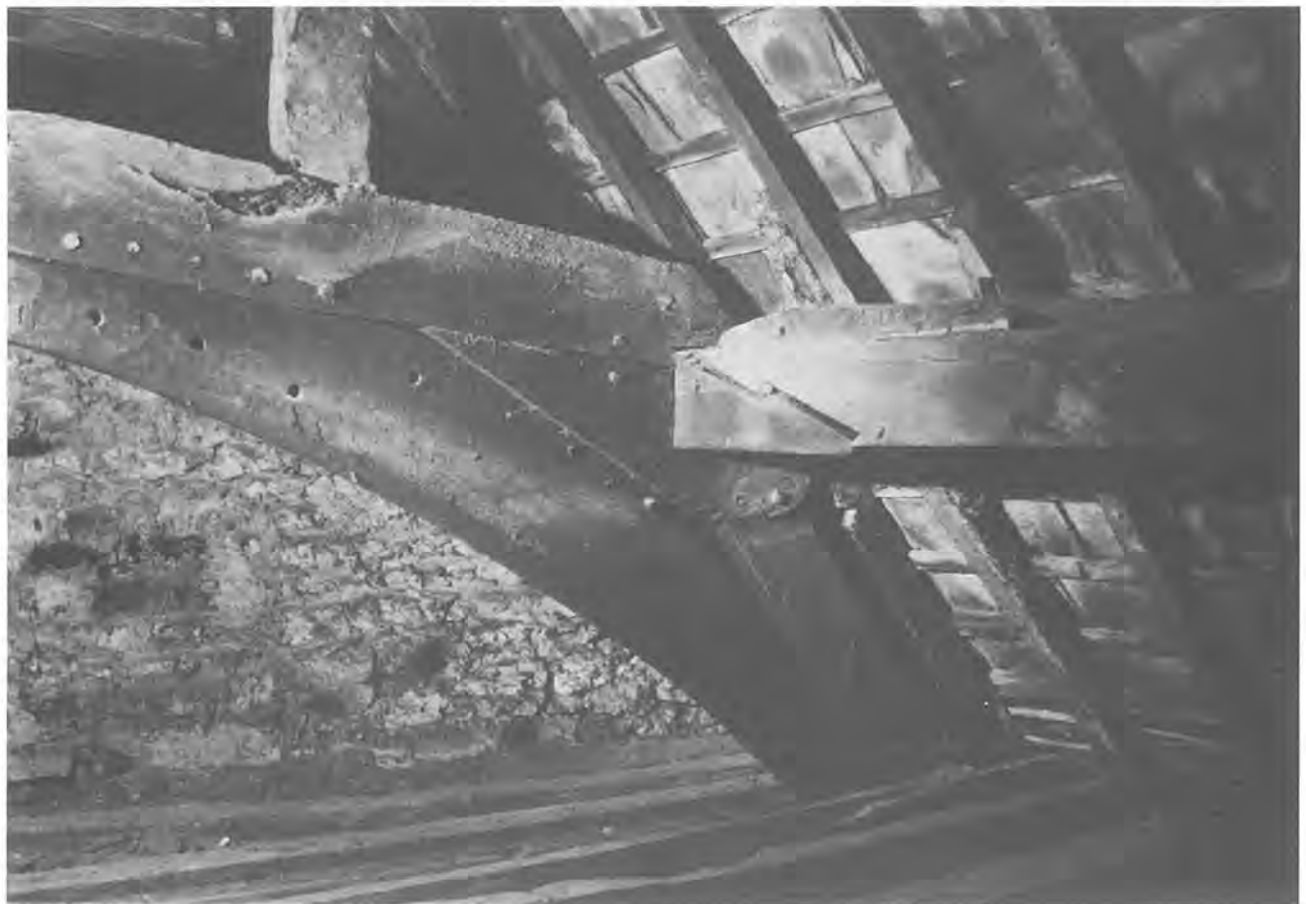
Figure 6. Hall House, Newland. West face of truss °/// and plate scarf.
