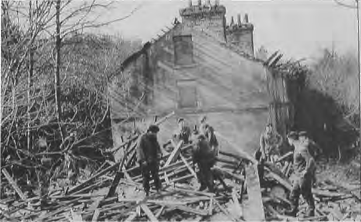
Figure 6: Demolition of Maryland March 1964 (Dorset Wildlife Trust Brownsea Archive)
