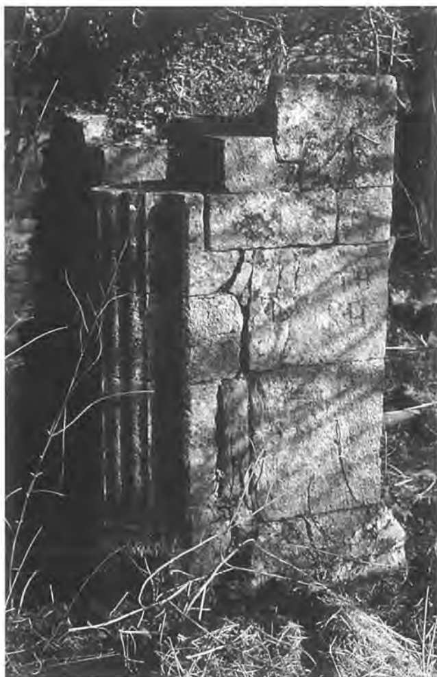
Figure 4: The south-east corner of the porch of the Old Church. The ashlar blocks of this section have been cut in a curious fashion that suggests that the porch was re-assembled here after being removed from a previous site. The mass dial is 'scratched' upon the uppermost surviving stone (Iain Hewitt)
