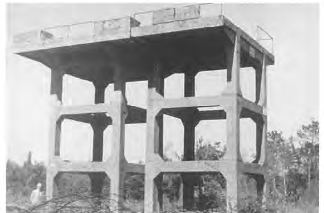
Figure 2: Two anti aircraft positions were built to the west and north-west of the factory site. Each consisted of a cannon mounted on one of a pair of towers. The other tower carried the director for aiming the gun, the two being separated to avoid vibration upsetting the director
