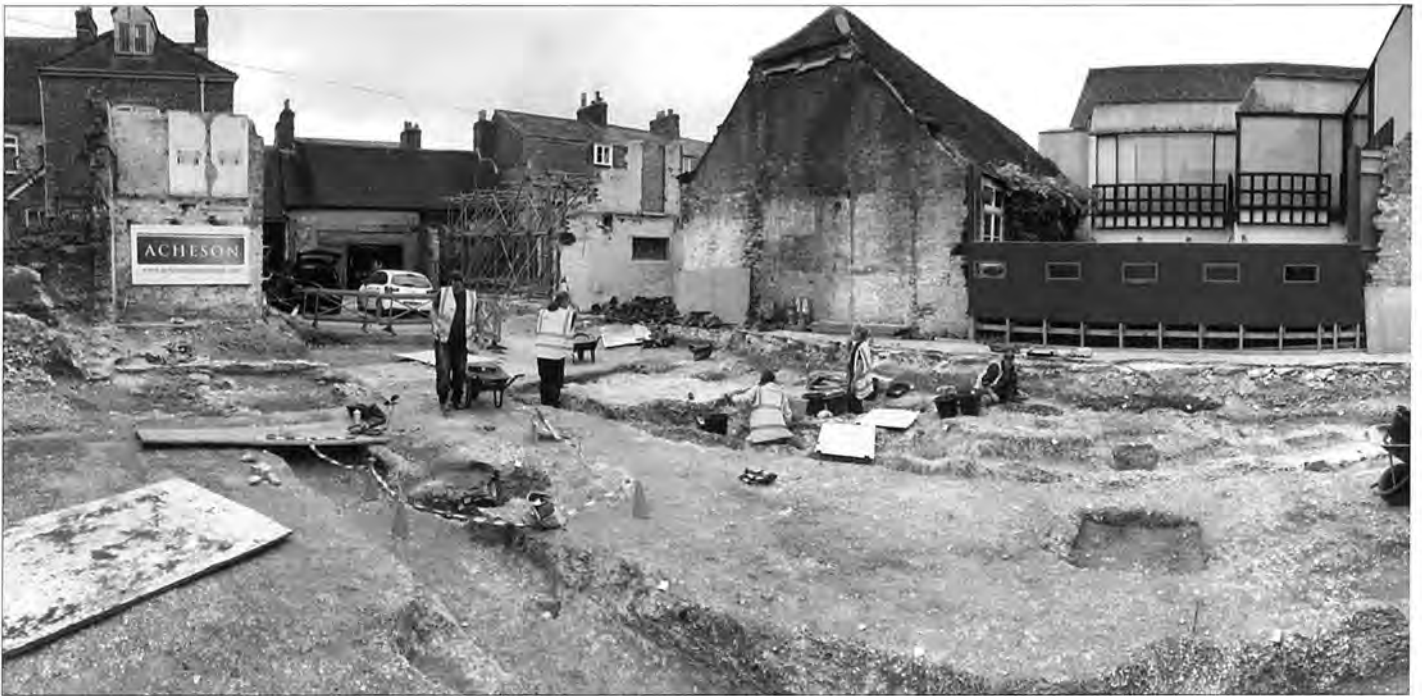
Figure 5: A panoramic view of the site under excavation
