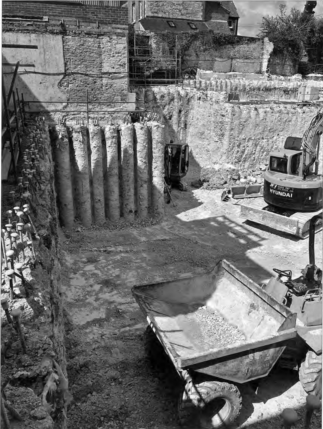
Excavating the basement
