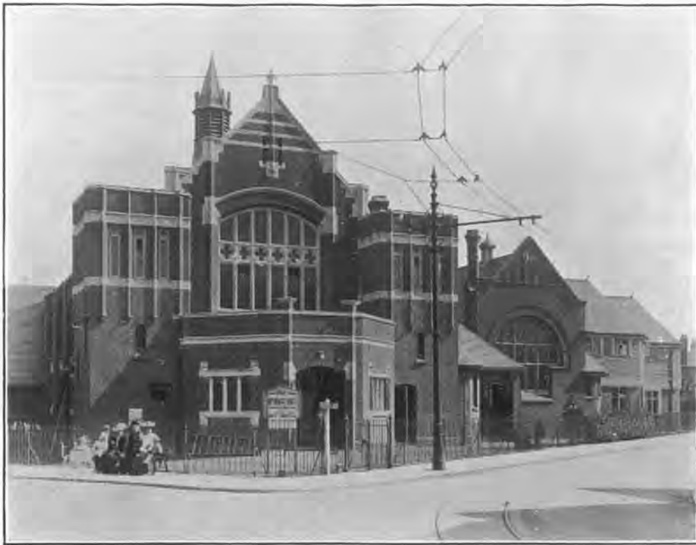
Charminster Road Congregational Church, Bournemouth, Completed and Opened, September 13th, 1905.
