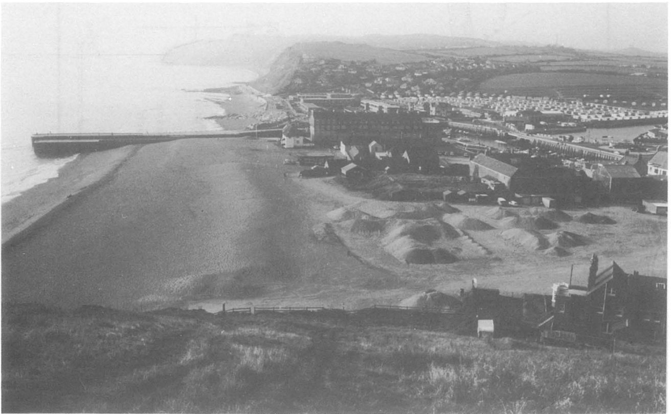
Plate 1. The western end of Chesil Beach at Bridport Harbour (West Bay), looking towards Eype. The harbour breakwaters have intercepted westward-drifting small pebbles to form a prograded beach. Beyond them the beach is long and narrow, and cliff recession has been halted by the building of an esplanade.
