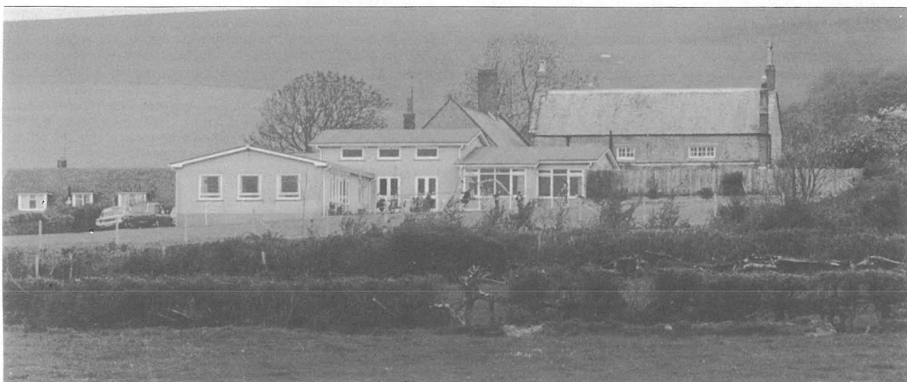
Plate 2. The School viewed from the south in 1984. The modern buildings (1968) are in front of the 1878 schoolroom. The master's house (1774) was built like a typical large farmhouse of the period with two ground floor rooms, two first floor bedrooms and two attic bedrooms. Originally there were no windows on the south side.
