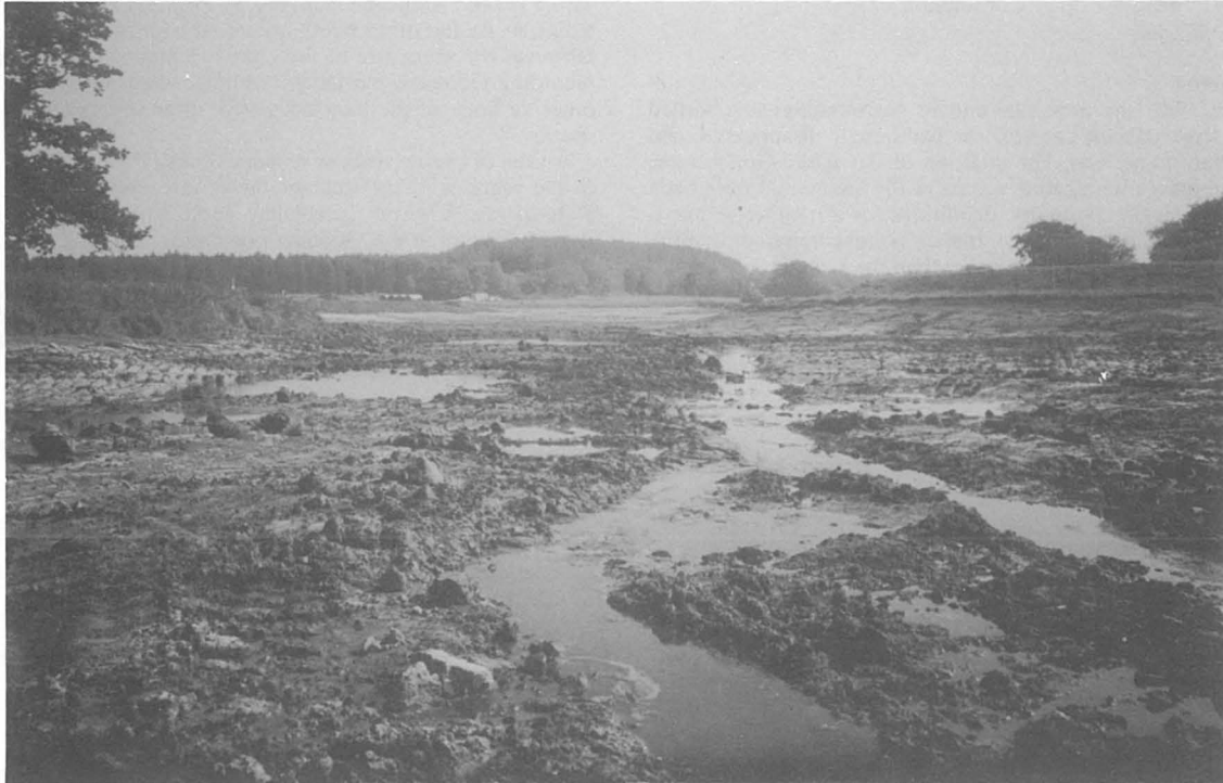
Plate 3. Excavation of Lake by King's Farm 1985.
