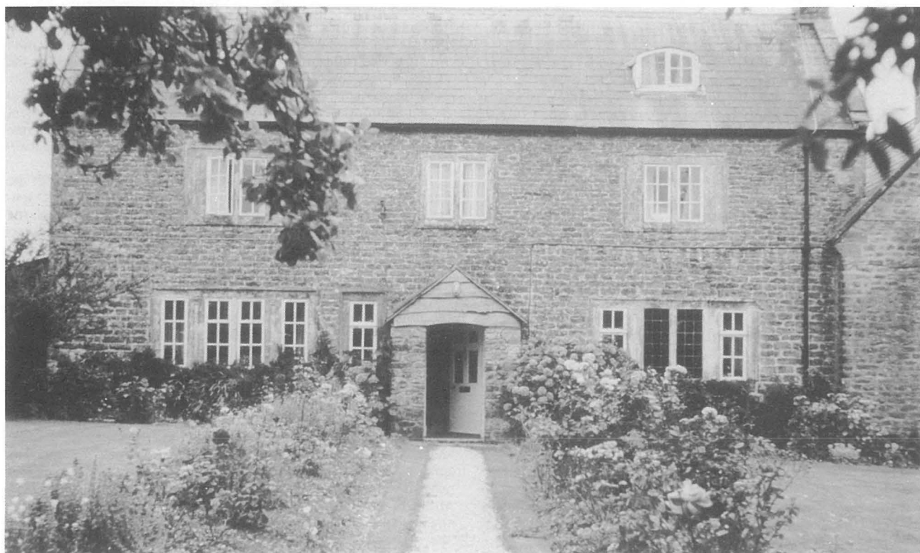
Plate 3. The north elevation of the house in 1970. The old schoolroom is on the right. All the windows still have their Ham Hill stone mullions but only two sections of the original leaded lights have survived.
