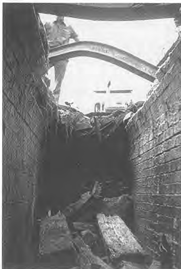
Plate 1 Motcombe: Hawker's Hill Brickworks: Underground fire tunnel, probably 19th century, revealed by digger in the 1980s. The tunnel was c. 10-12ft long and c. 8ft high.
