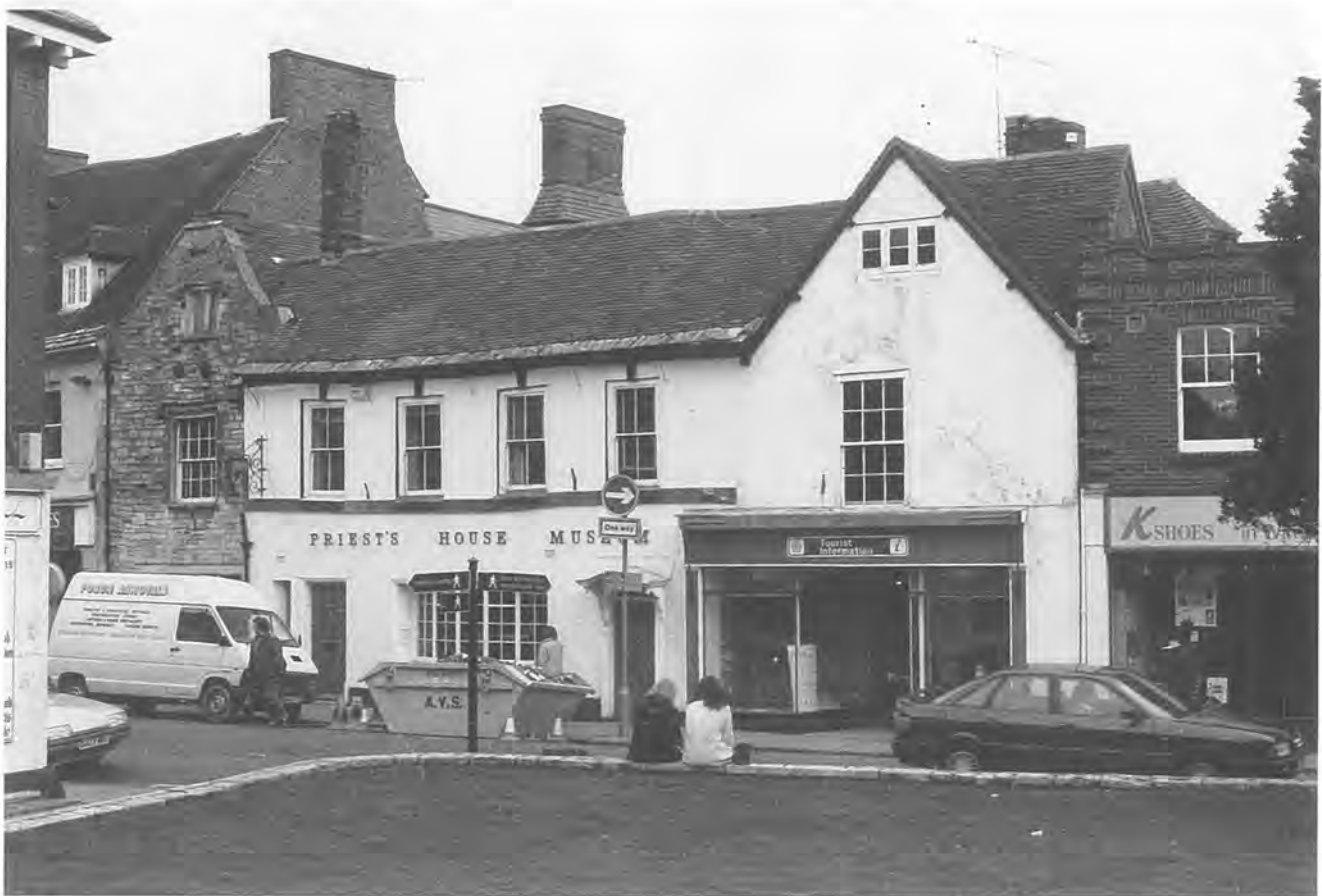
Plate 1:- 29 High Street from the West: Pre-Renovation.
