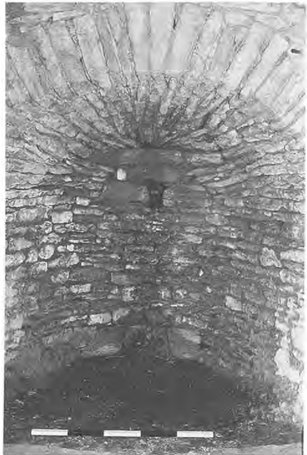
Plate 6. Stone draw arch, recess, poking hole and draw-hole at Old Quarry limekiln, Longburton. July 1993. Scale: 1 metre.
