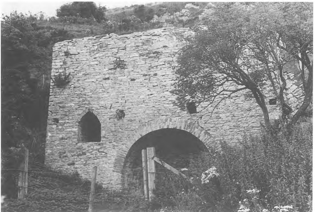
Plate 9. Bucknowle limekiln at Church Knowle, showing the brick draw arch and the lime-burner's bothy window. 1988.
