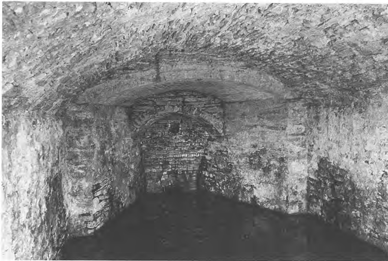
Plate 5. Double draw arches and a high quality of building seen at the Whitmore Coppice limekiln. The site was flooded on the day of the photograph. June 1993.
