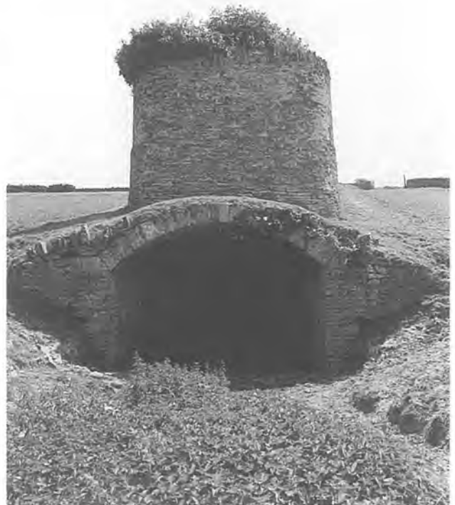
Plate 4. Whitmore Coppice limekiln from the north, showing the unusual tunnel approach to the draw arch area. June 1993.
