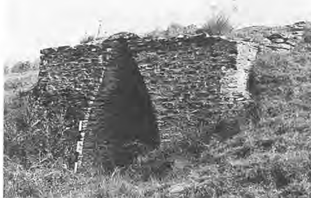
Plate 2. New Lane, Swyre. A small pointed arch Type C limekiln. July 1993.
