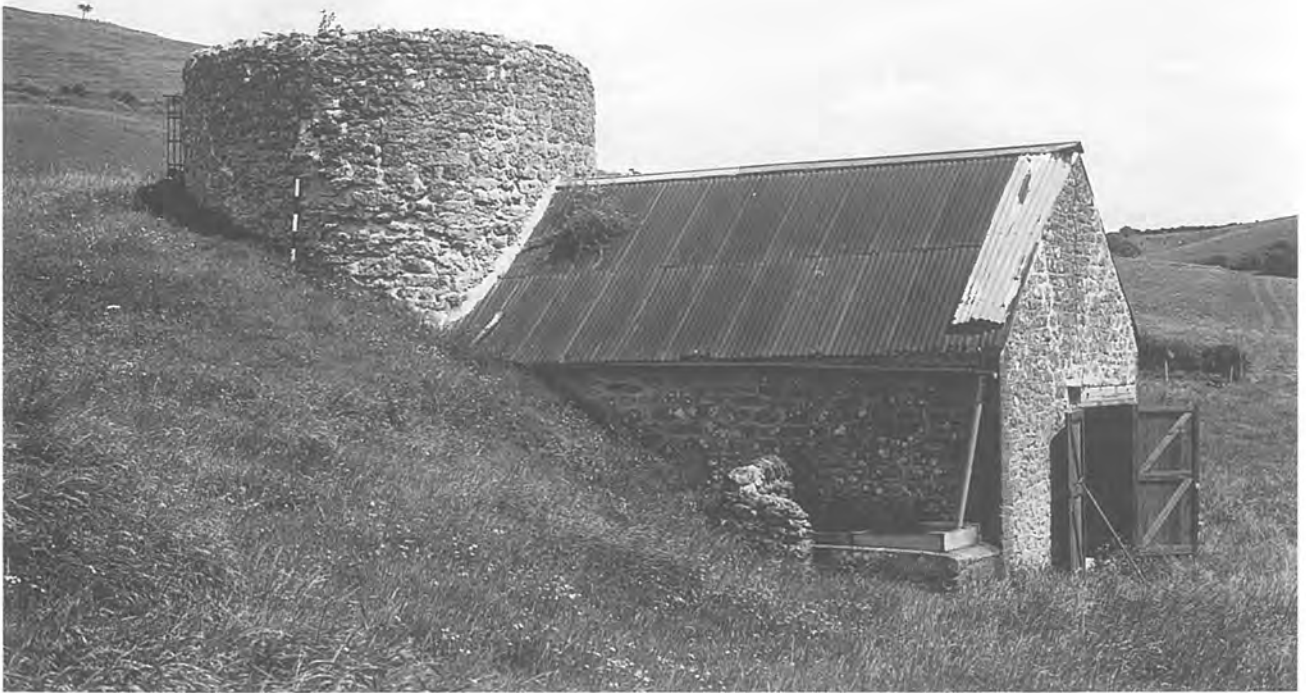
Plate 8. Bell House limekiln, Lodgers: a well preserved limekiln and lime shed viewed from the west. July 1993. Scale: 1 metre.
