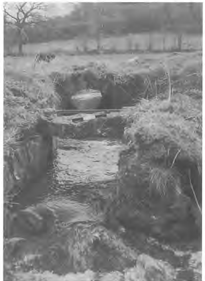
Plate 1 Sluice No. 2 from north-west side, showing bridge with voussoirs.
