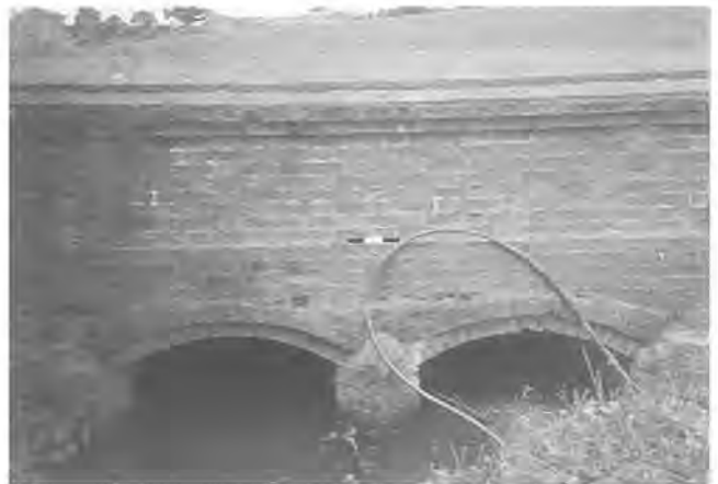
Plate 3. Brick bridge near Whittings Farm.
