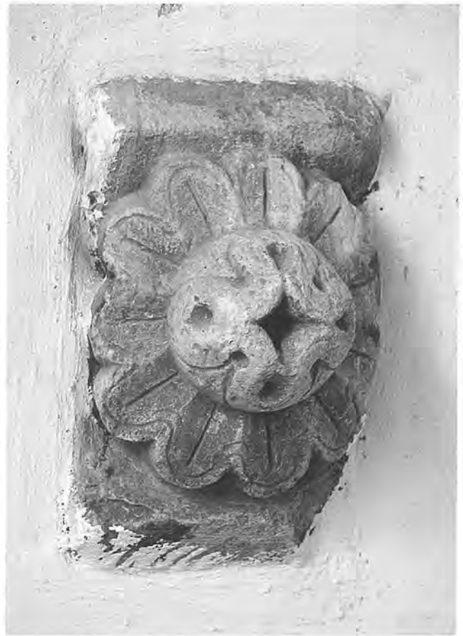
Figure 37: Maiden Newton, Romanesque rosette corbel reused in south wall of south transept (Photo: M. Thurlby)
