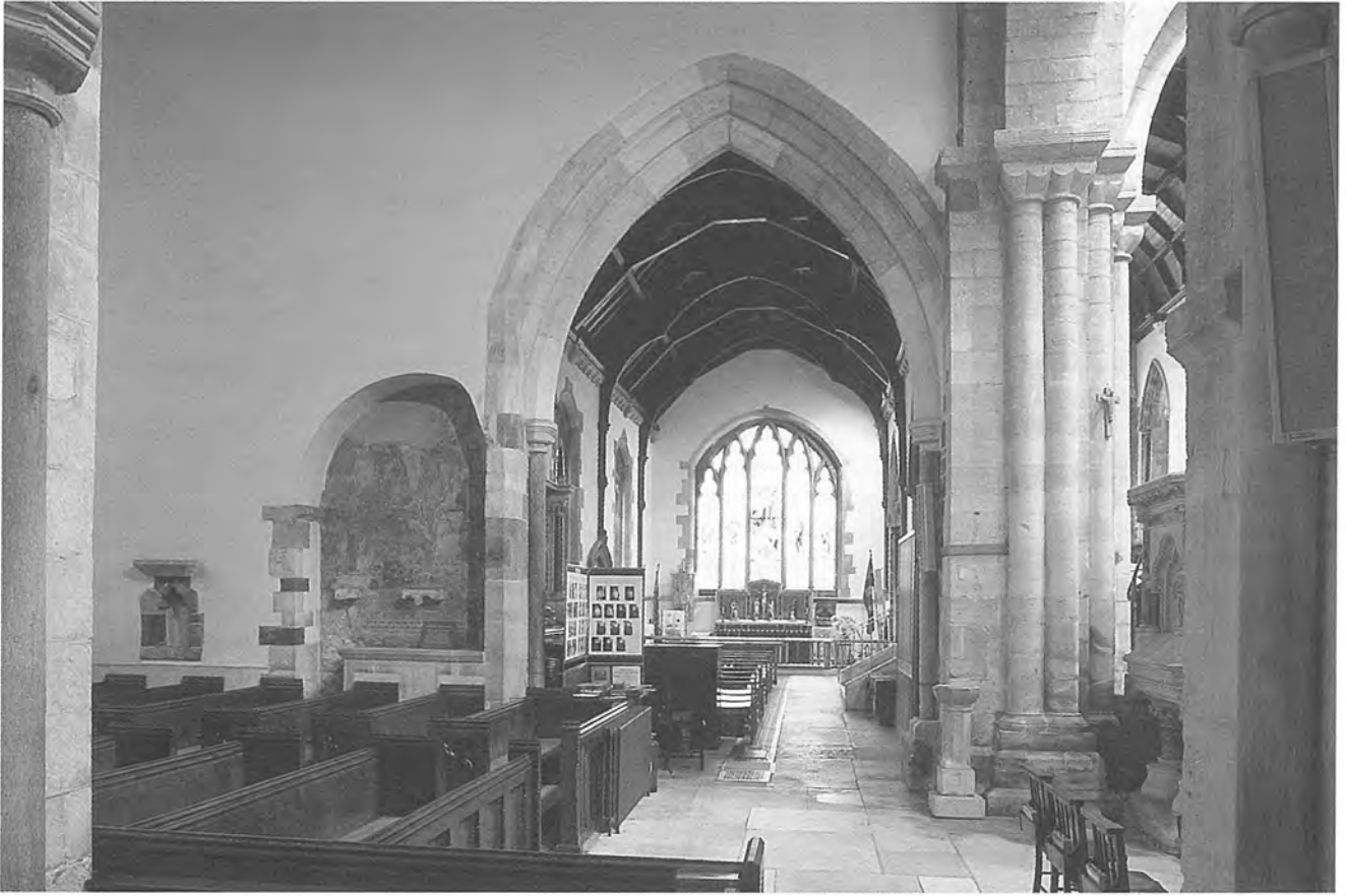
Figure 2: Wimborne Minster, north transept, interior to east (Photo: M. Thurlby)
