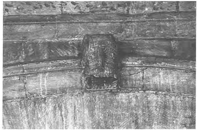
Figure 17: Sherborne Abbey, north crossing arch, detail south (Photo: M. Thurlby)
