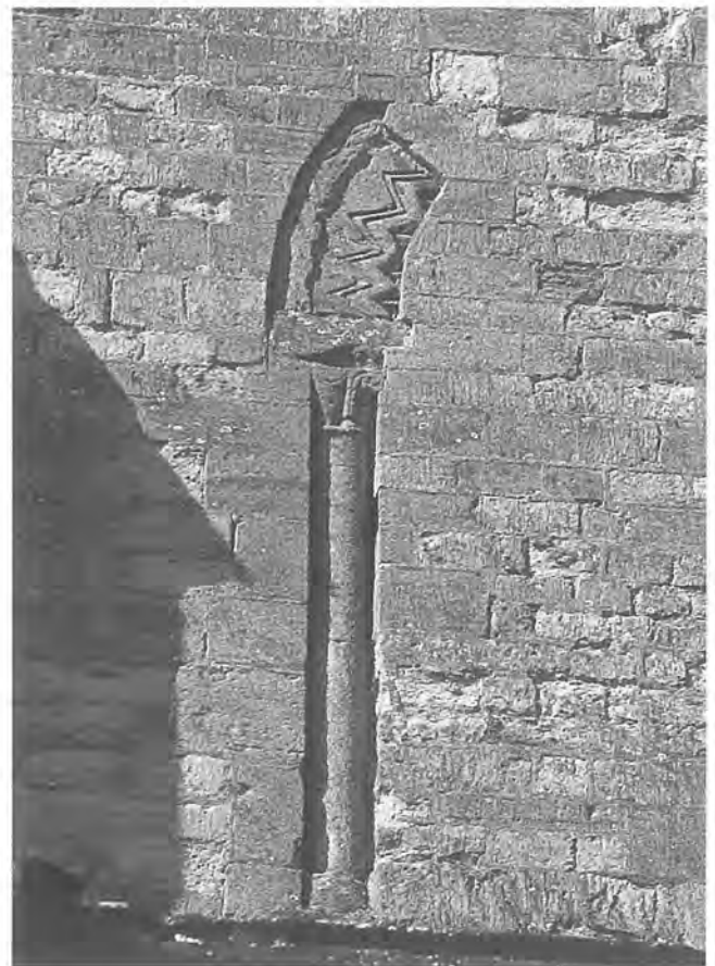
Figure 10: Sherborne Abbey, south transept, east wall, detail of former clerestory window (Photo: M. Thurlby)
