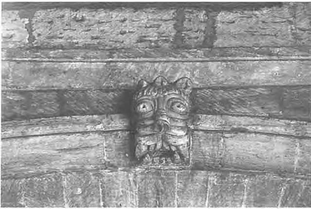
Figure 16: Sherborne Abbey, south crossing arch, detail north (Photo: M. Thurlby)
