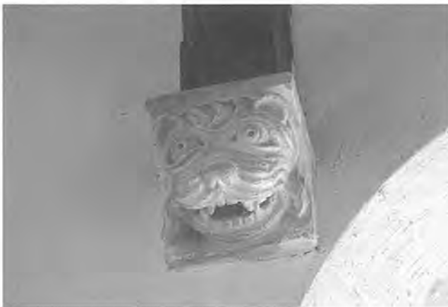
Figure 32: Maiden Newton, Romanesque corbel, re-used as nave roof corbel N2 (Photo: M. Thurlby)
